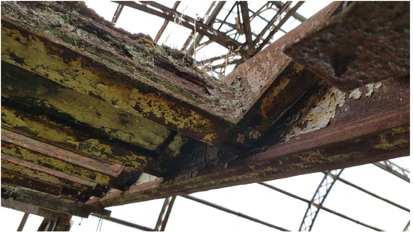
25 – Steel stairs have been damaged but the remaining steel is in reasonable condition and they could be repaired
