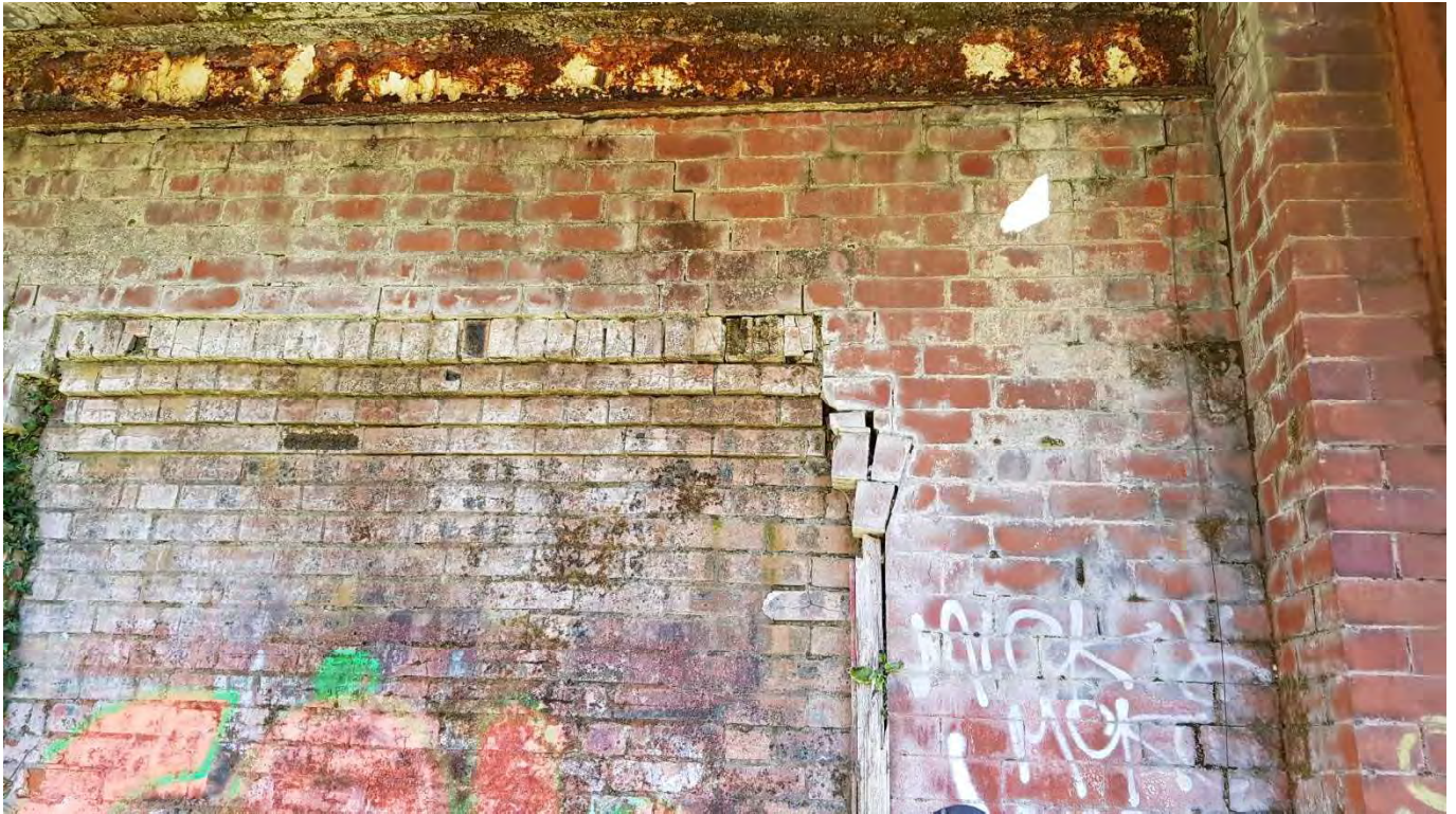
46 – Infill of original opening shows signs of failure near the bearing end
