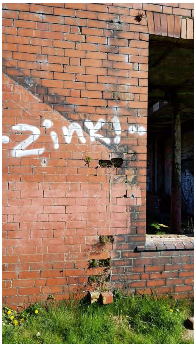
38 & 39 – Missing bricks and small cracks up masonry jamb and corner deterioration and movement of the upper panel
