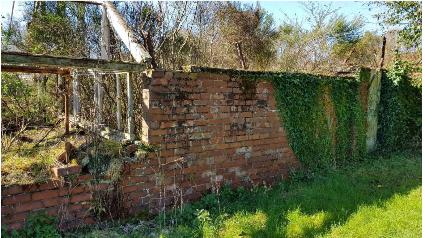
62 – View of west end of north wall where it becomes a freestanding boundary wall. Ivy growth and water ingress through the cope has caused deterioration in the brickwork
