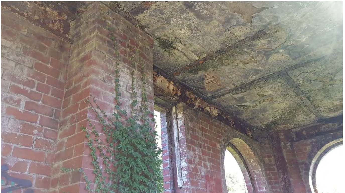
47 – Internal view of pier in good condition along with steel beams and filler joists
