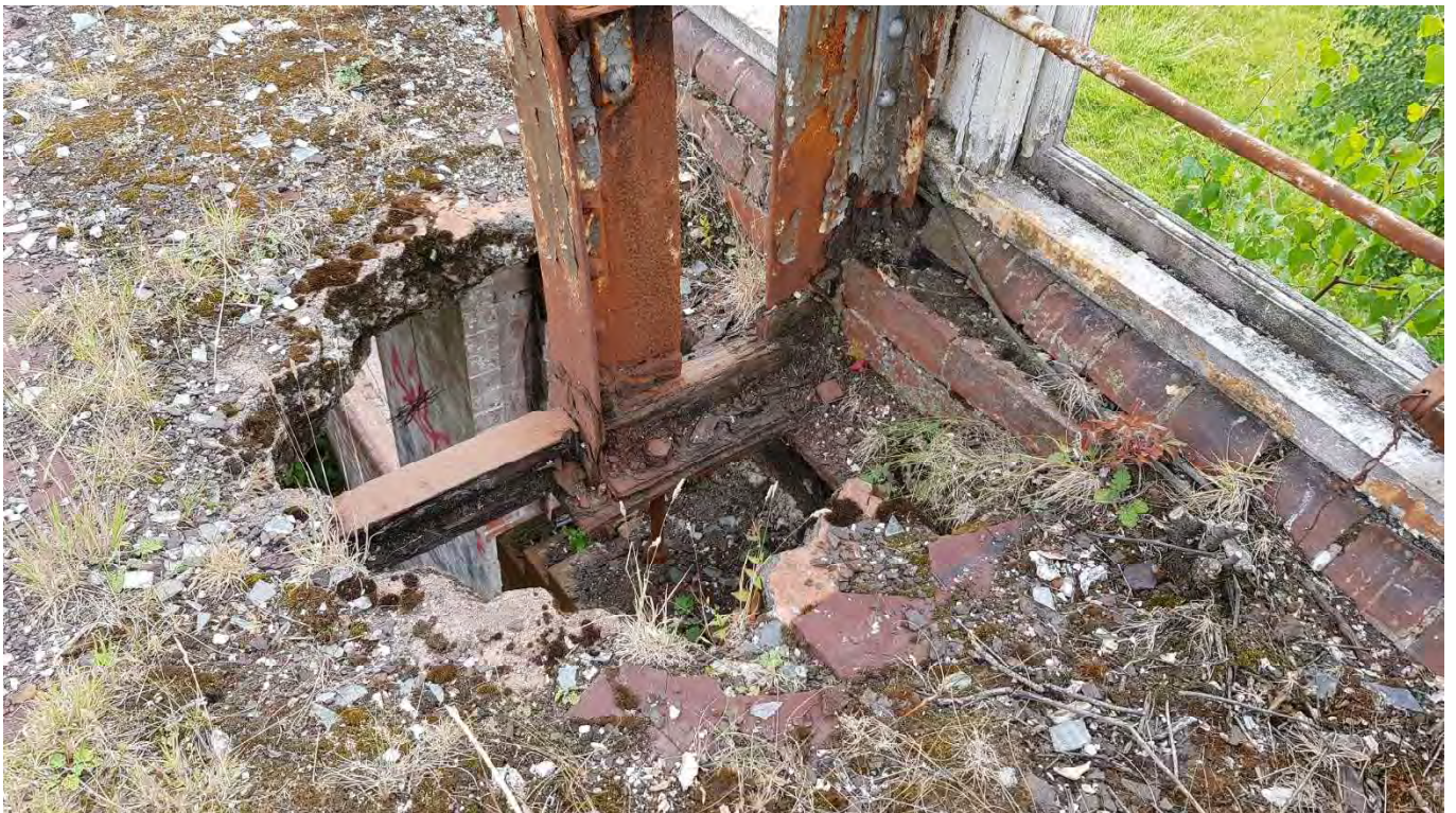
8 – The opened-up lattice frame base to the south-west of the Main Hall, showing some delamination and loss of rivets/bolts at slab level
