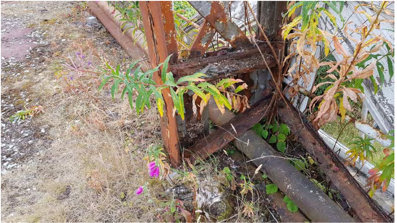
7 – Base of one of the lattice frames on the west elevation showing the localised corrosion of the lower level angles
