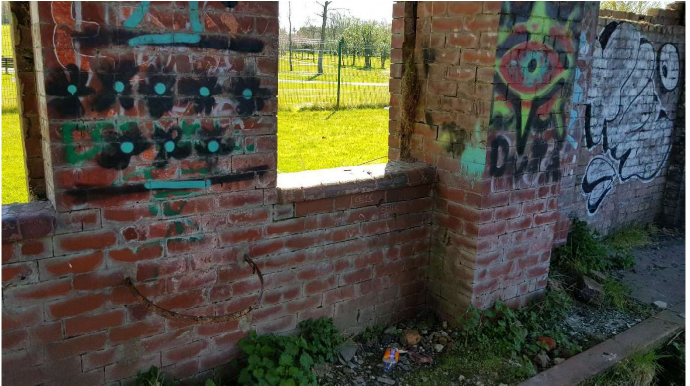
48 – Masonry panels on the east elevation which are in reasonable condition structurally
