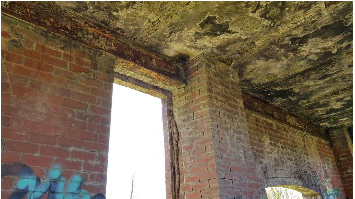
49 – Root growth at window jamb has caused outwards movement of the outer pier masonry
