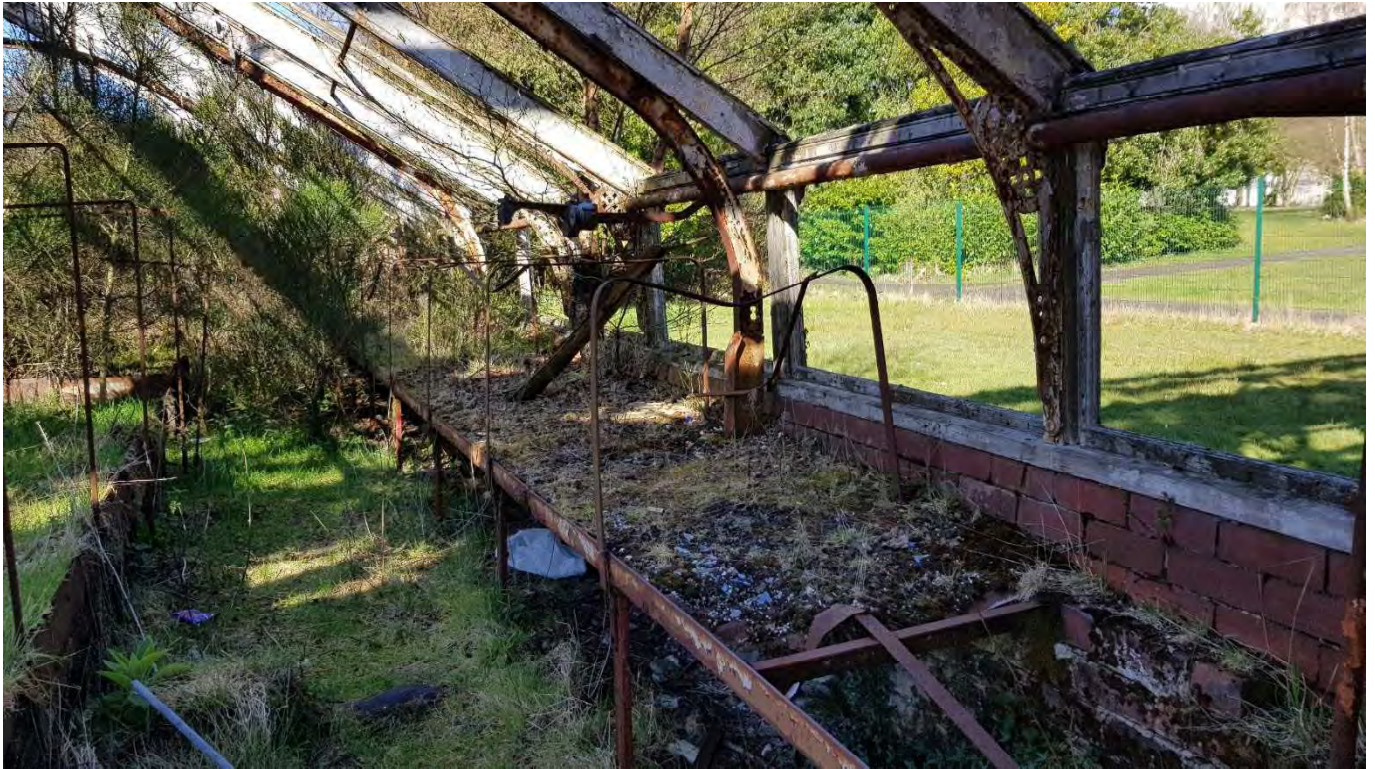
66 – View to north showing the condition of the timberwork which might be able to be re-used and saved
