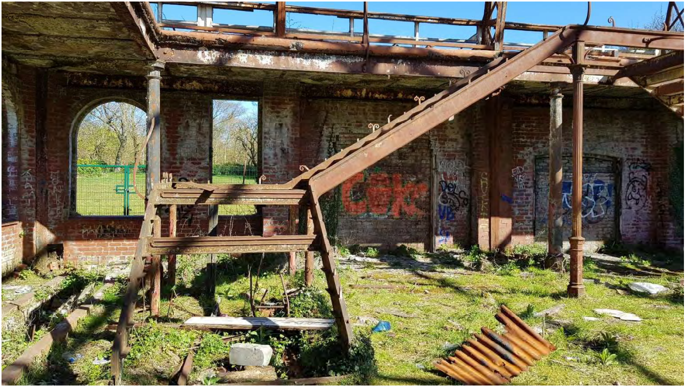
27 – View of steel stairs to north, which again can be repaired
