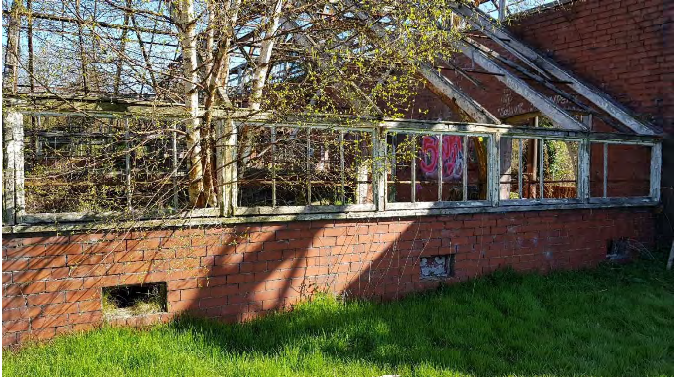
69 – Vegetation growth through the structure needs to be removed and the existing framing re-used
