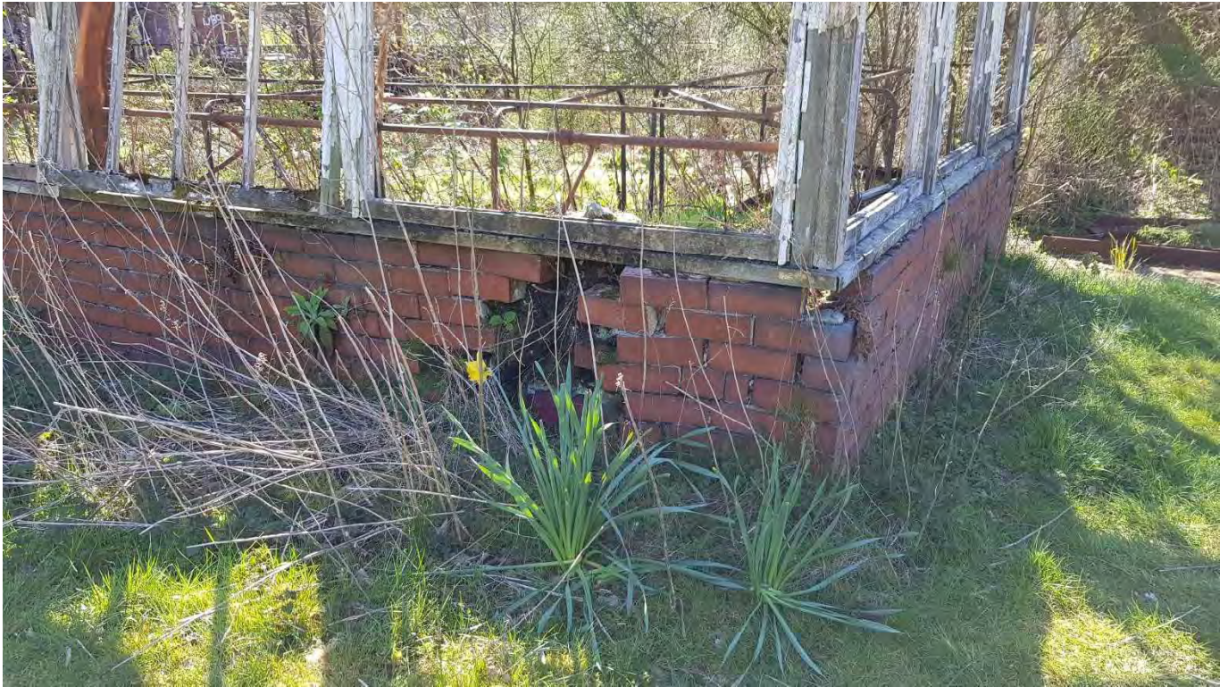
72 – Partial collapse of masonry at north-west corner which will need to be rebuilt
