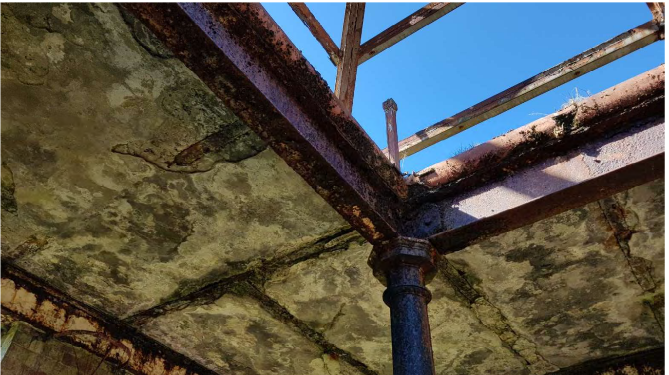
24 – Corroded steel beams at the corner which will need re-painted, but are intact
