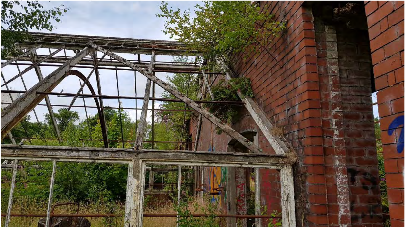
74 – Connection of south glasshouse to Main Hall walling with vegetation in the masonry jointing and some poor connections of the original rafters
