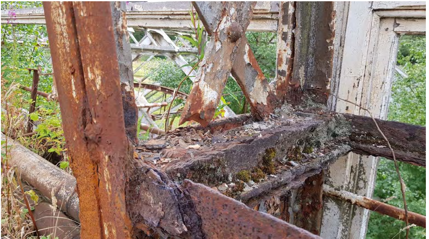
12 – View of one of the worst corroded angle frame connections with severe deterioration of the steelwork locally
