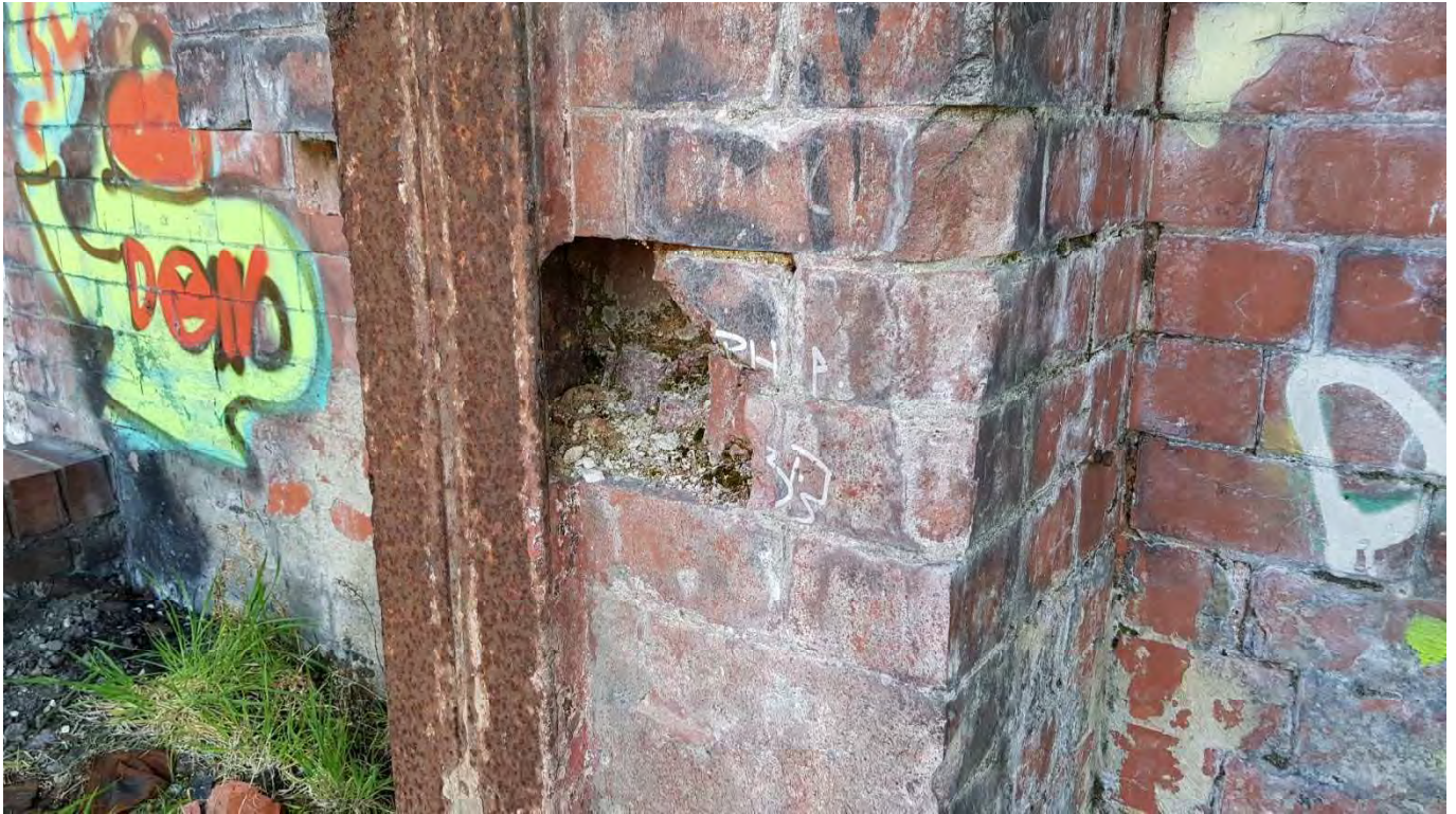
52 – Localised opening-up at stanchion showing surface corrosion
