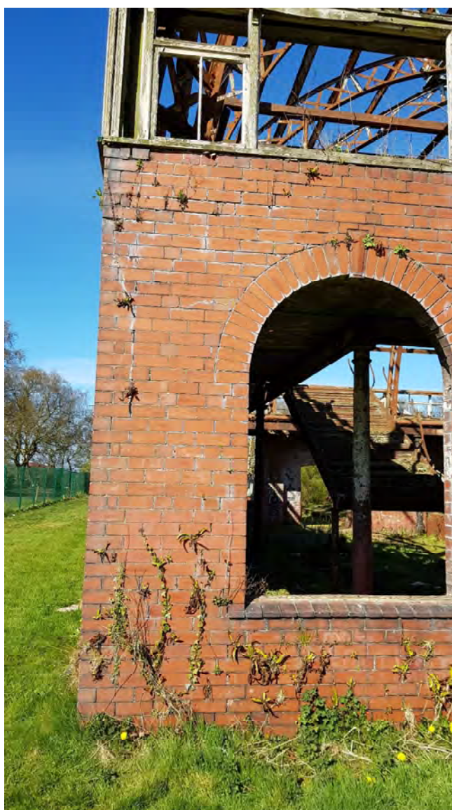
38 & 39 – Missing bricks and small cracks up masonry jamb and corner deterioration and movement of the upper panel
