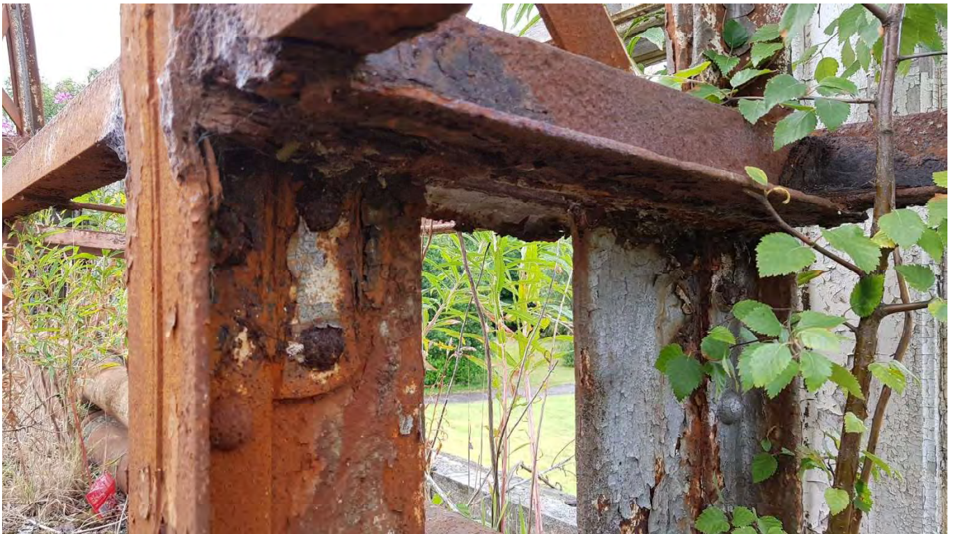
14 – Close-up view of lower frame connection with more deterioration to rivets
