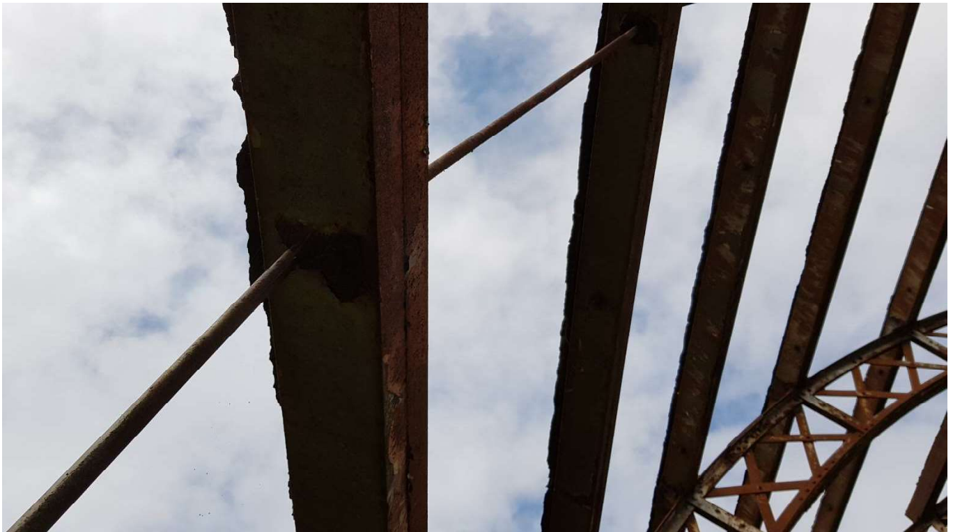
6 – Similar to Photo 5, the corrosion of the main purlins on the north elevation is severe, but the anti-sag rods appeared to be in reasonable condition
