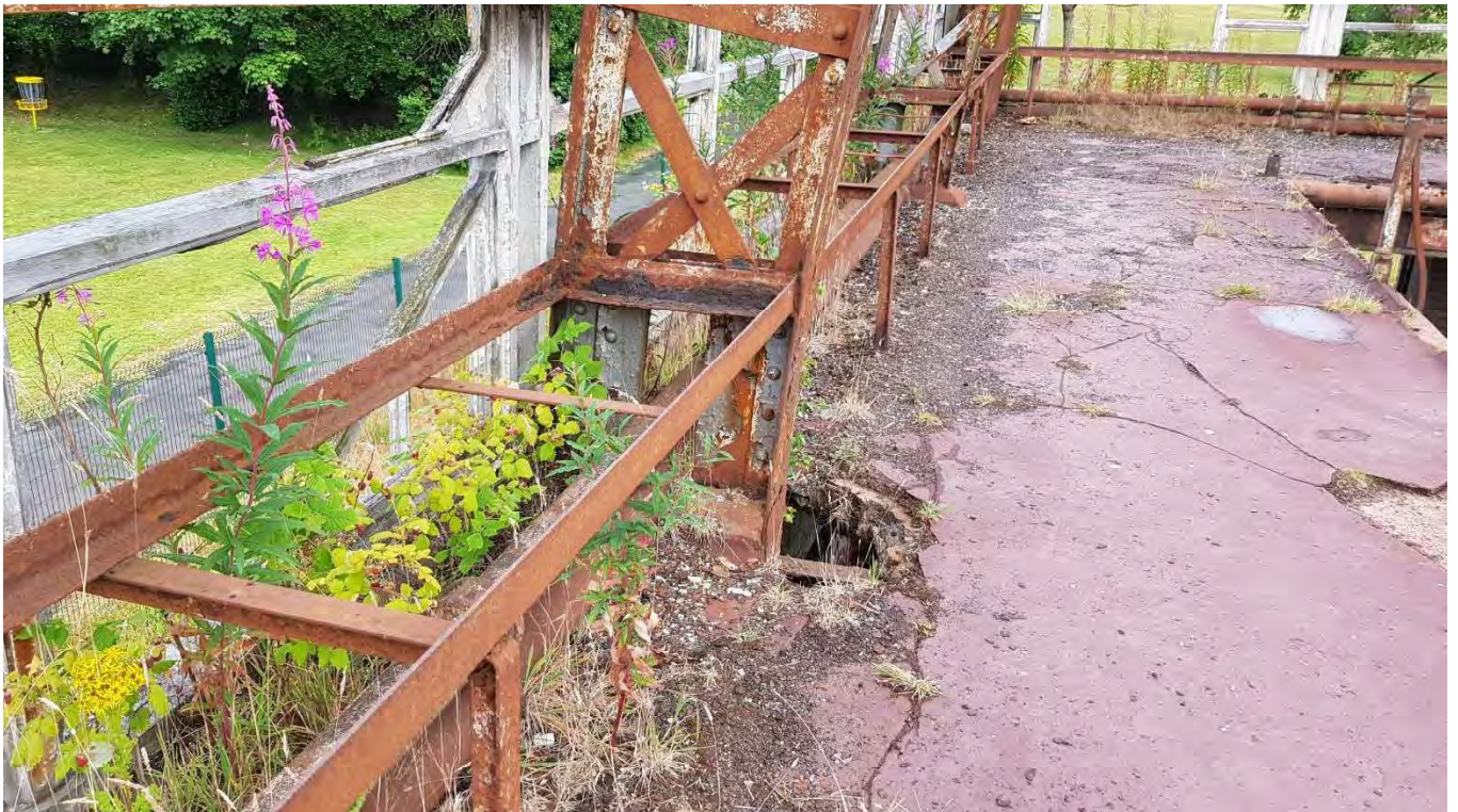
10 – View along north balcony with cracked finishes to slab and the original table framing. Some original paint finishes are still shown on the steelwork
