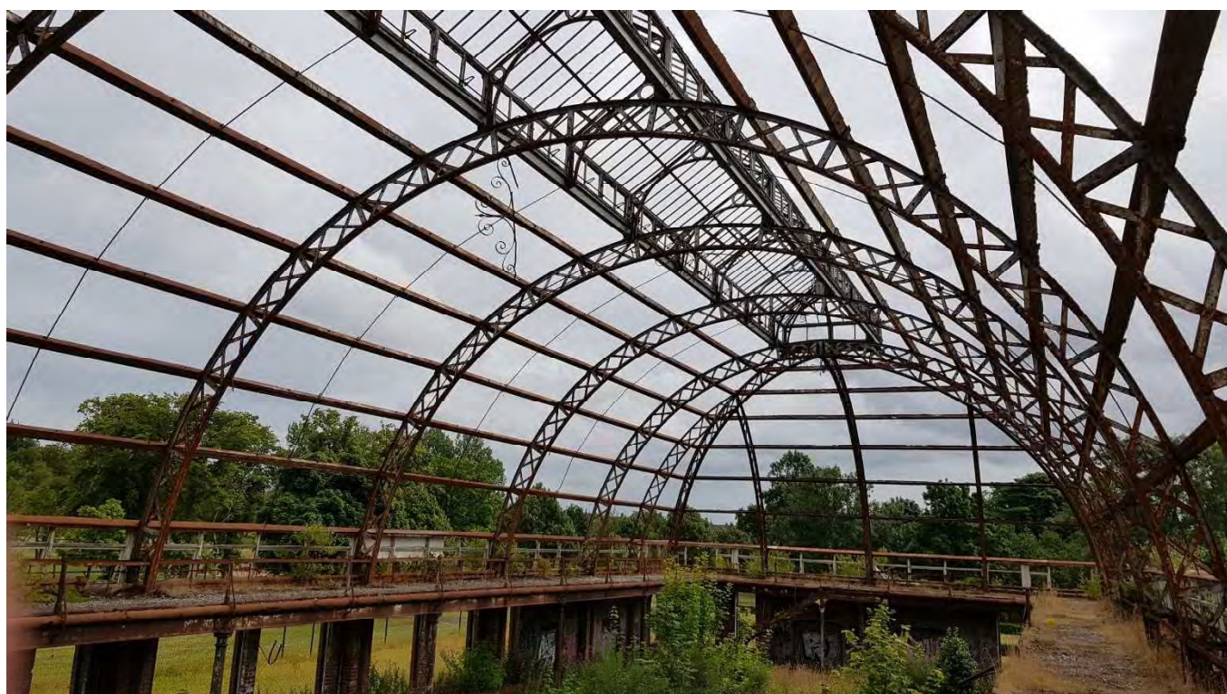
2 – View to south-east showing the regularity of the main lattice frames and the 'hanging' steel bracket
