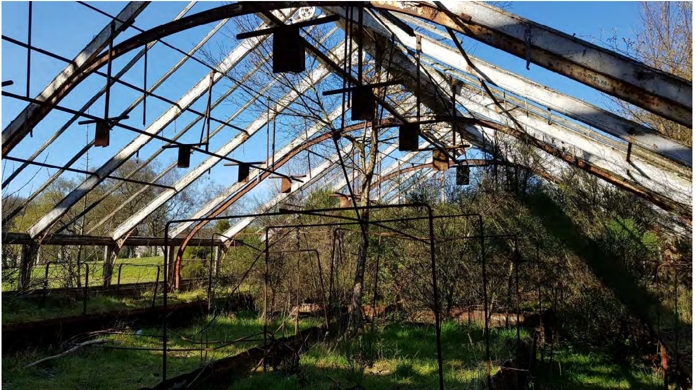
64 – View along glasshouse showing general geometry has been maintained but needing re-set
