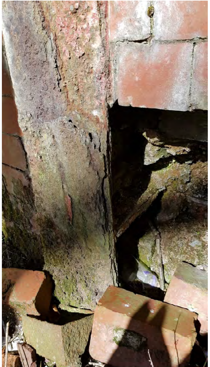
44 & 45 – Internal view of embedded stanchion and localised delamination at opened-up section
