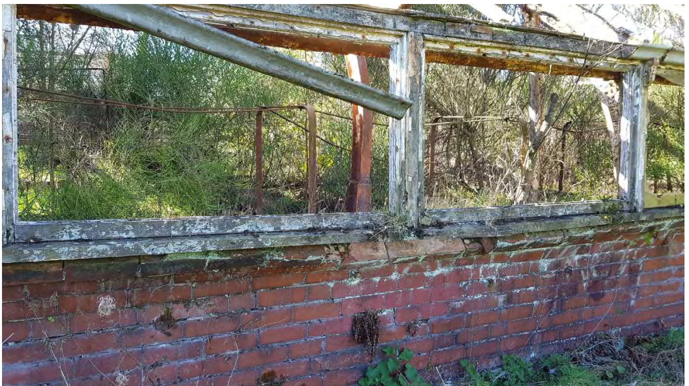
61 – Close-up view of failed wall section with the upper brickwork rotated outwards dramatically. Note the steel 'hoop' within the glasshouse is intact with minor surface corrosion
