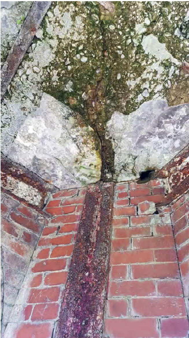
44 & 45 – Internal view of embedded stanchion and localised delamination at opened-up section
