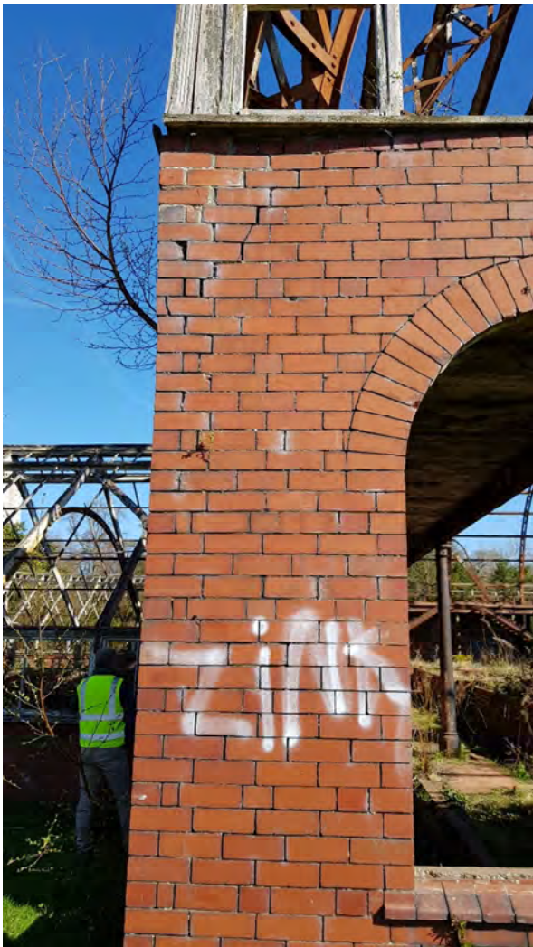
32 & 33 – View of south-west corner vegetation and cracking/movement and some missing bricks
