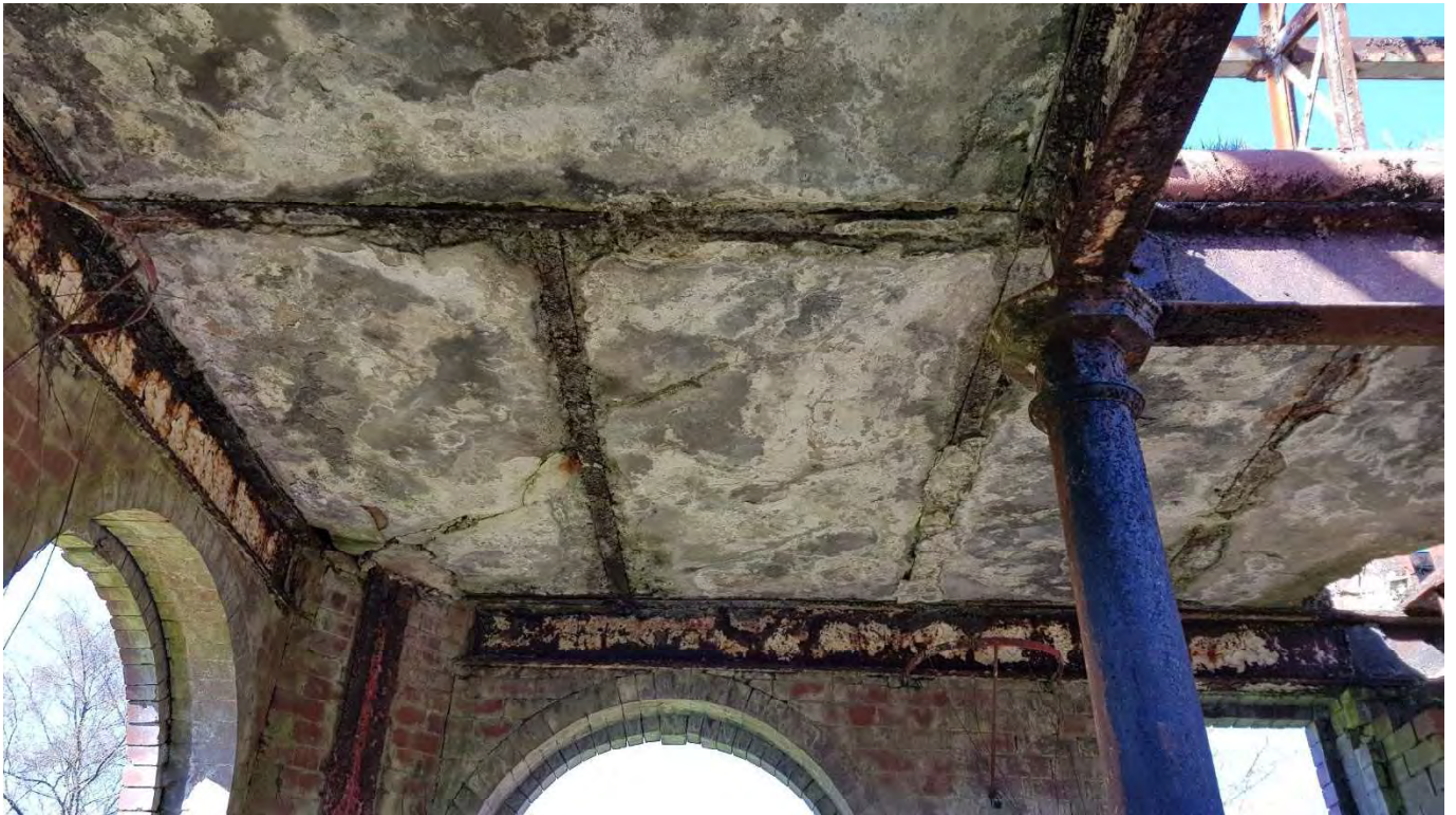
21 – Underside view of balcony slab and steel edge beams and cast iron column. Edge beams still have paint remnants and although surface deterioration on filler joists and concrete, all can be repaired
