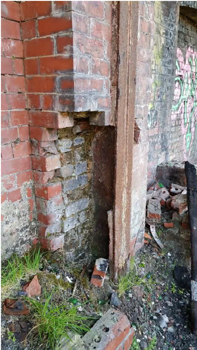
50 & 51 Deterioration or opening-up at internal stanchion base showing corroded but serviceable steelwork in the temporary case. Masonry deterioration to be repaired at main pier
