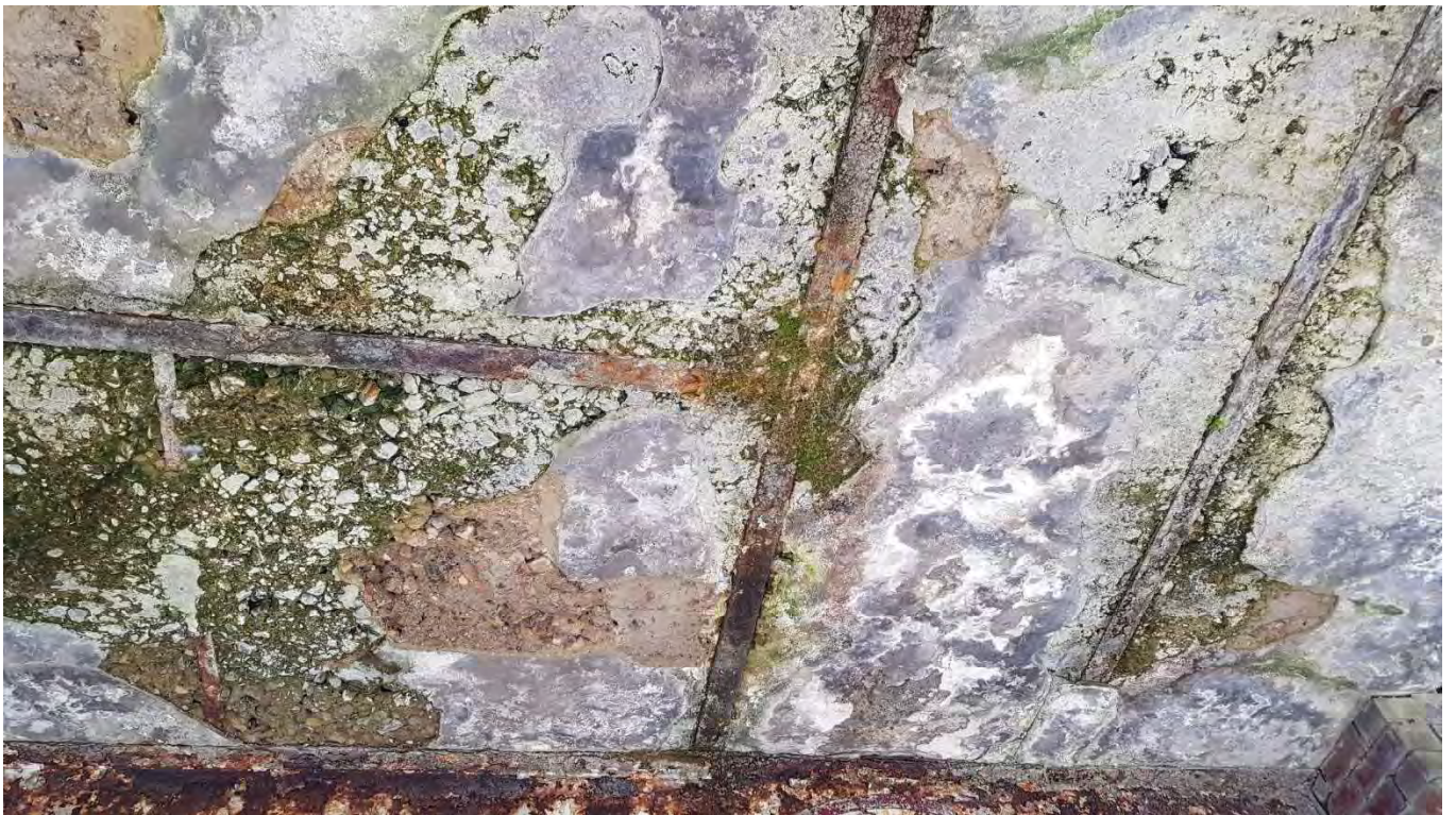
18 – View of underside of balcony showing filler joists with some corrosion and some spalling of the concrete infill, but the structure appeared intact
