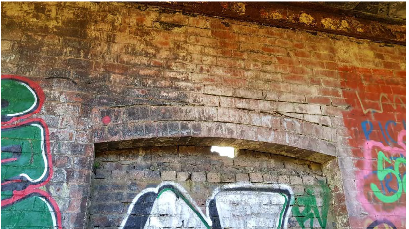
53 – Arch over opening appears to be intact and aligned properly
