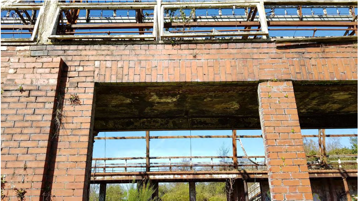
36 – Similar view showing the movement of bricks to the bearings of the main lintels
