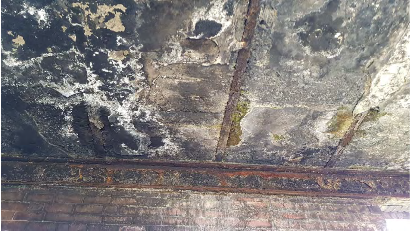
19 – Underside of balcony with corroded steel beam in the wall and some spalling in the slab
