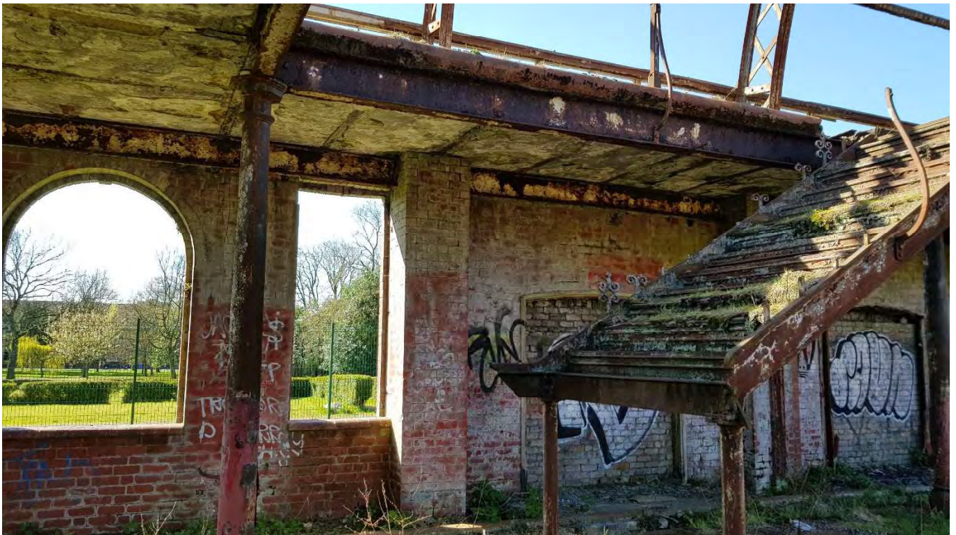
55 – View of stair at south end and cast iron column/steel ring beam around balcony
