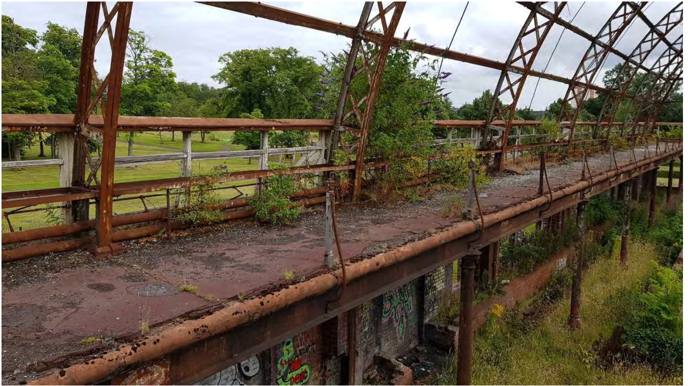
17 – West balcony showing missing balustrading and failed top surface
