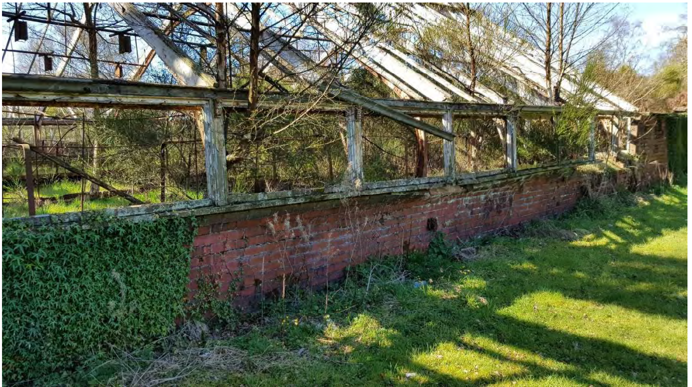
60 – View of partially-collapsed north wall which will need to be rebuilt
