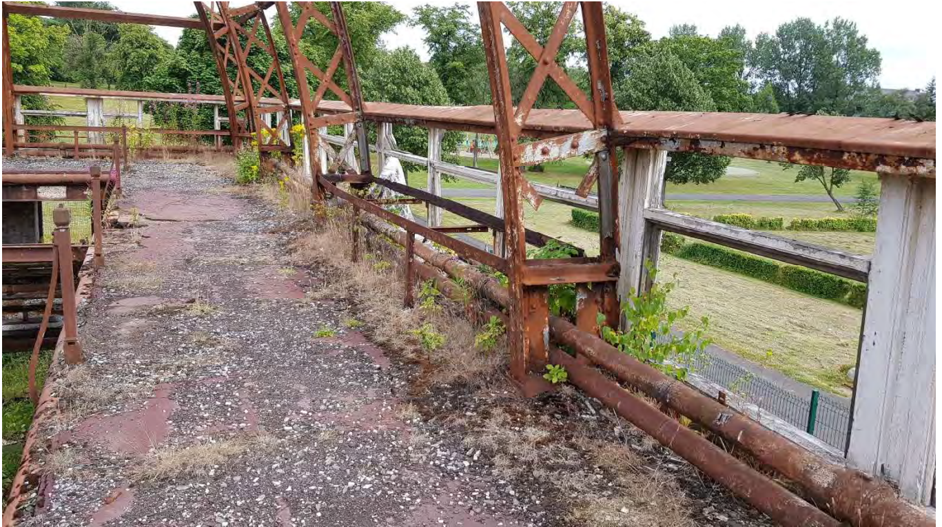
9 – View along the south gallery showing the condition of the floor surface and missing cross members in the main lattice frame
