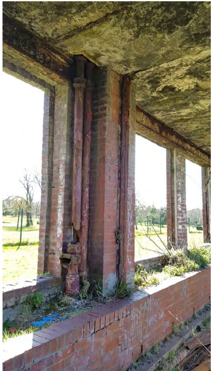
50 & 51 Deterioration or opening-up at internal stanchion base showing corroded but serviceable steelwork in the temporary case. Masonry deterioration to be repaired at main pier
