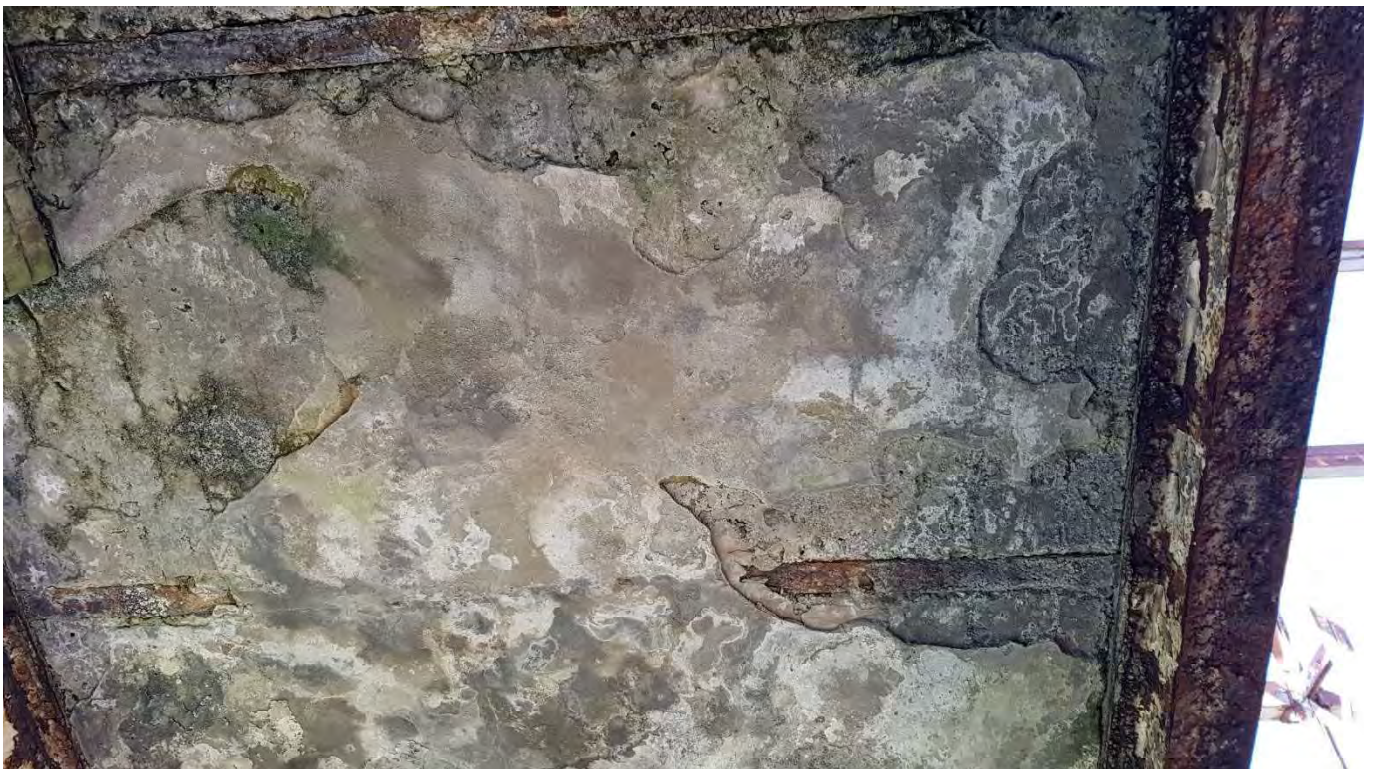
22 – Underside view of slab with more intact finishes and corroded steel support beam
