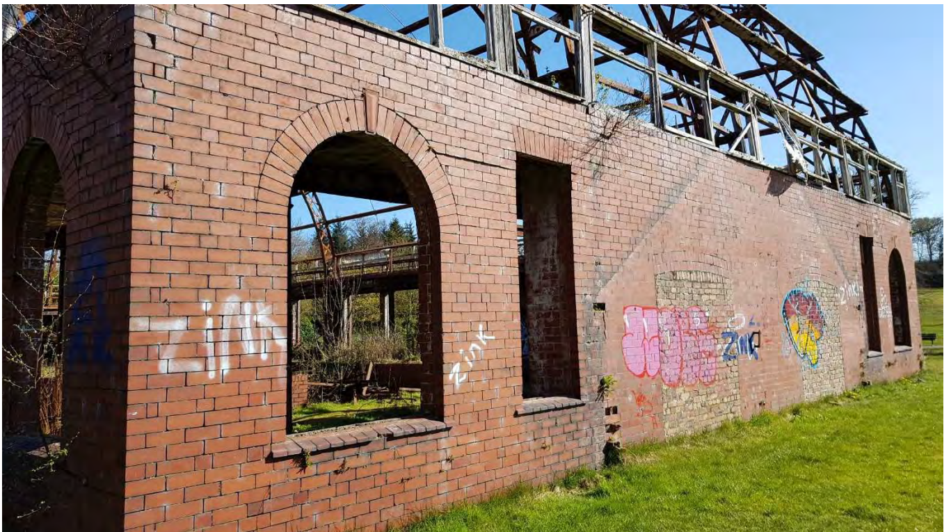
30 - View of north elevation showing the vestige of a northern glasshouse and bricked-up openings. Vegetation growth has rooted in the masonry mortar joints and will need to be removed
