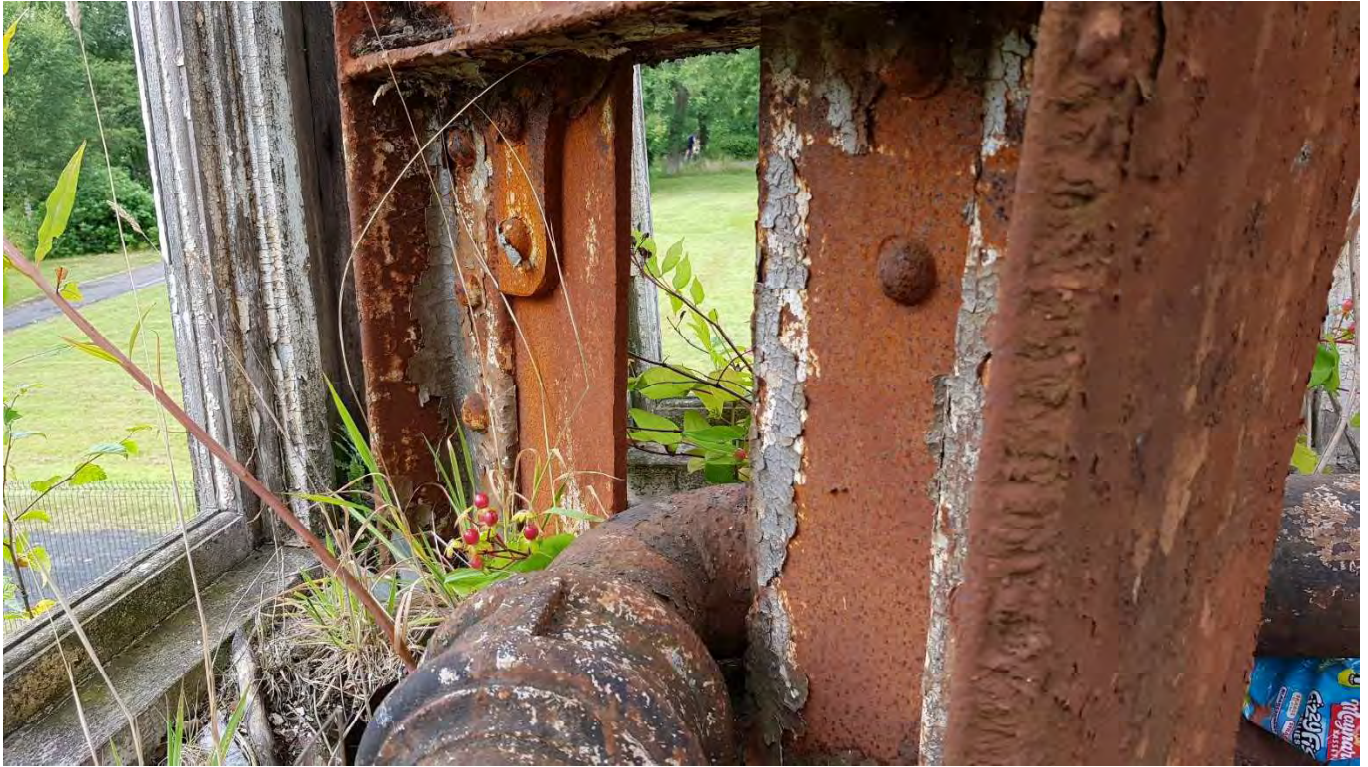
13 – View below the lower steelwork in the north-west corner with intact rivets and only surface corrosion
