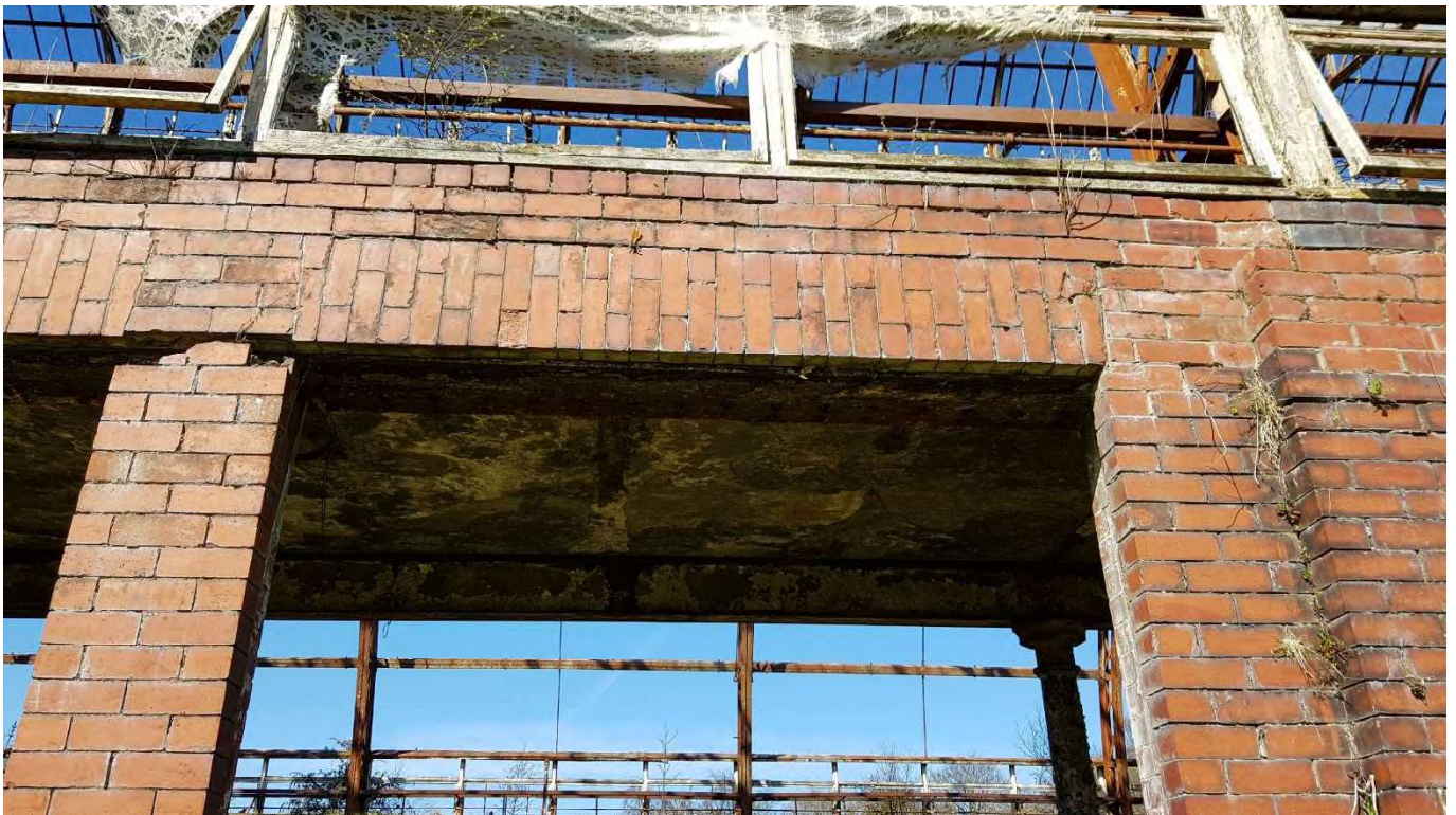
35 – Main flat arch with steel lintel behind showing localised jacking failure at the pier bearing
