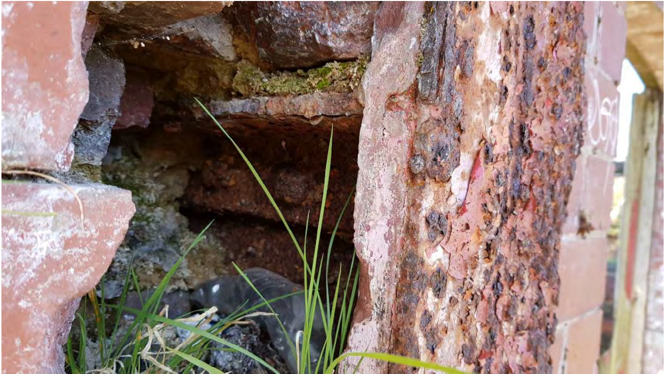
58 – Detail view of embedded steelwork showing some deterioration
