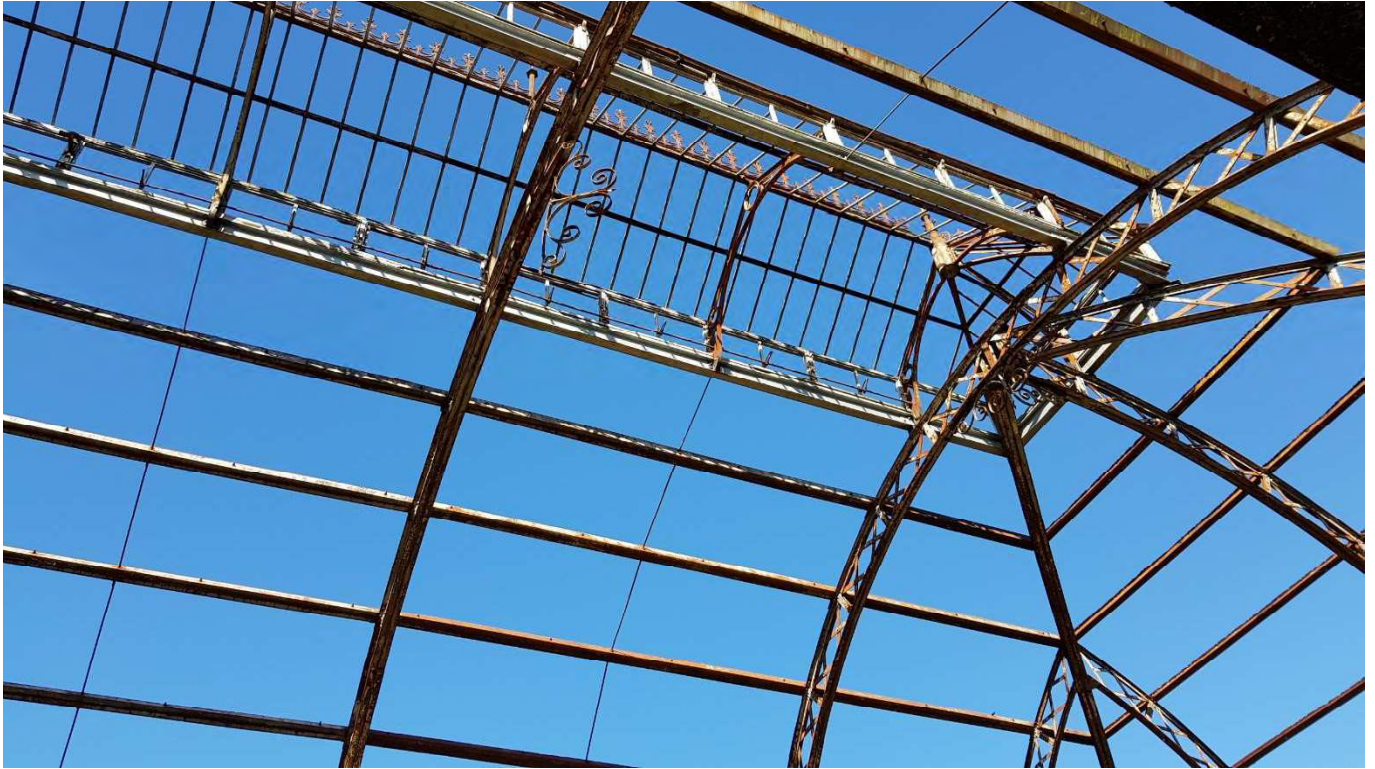
3 – View of 'hanging' bracket (looking north-west) and recently repaired cupola ringbeam
