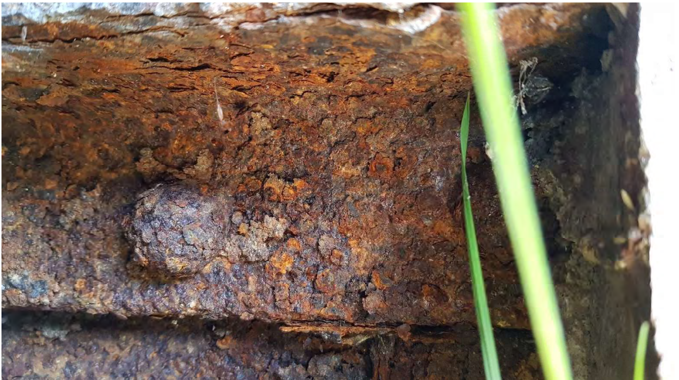
59 – Heavier corrosion including rivet heads which may need direct steel repairs for the longer term project
