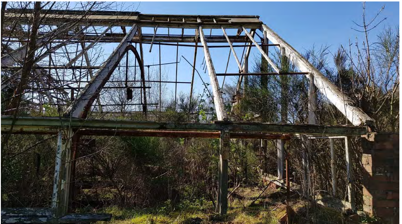
63 – View of west end of the glasshouse showing missing roof mullions and deflection in the upper purlins
