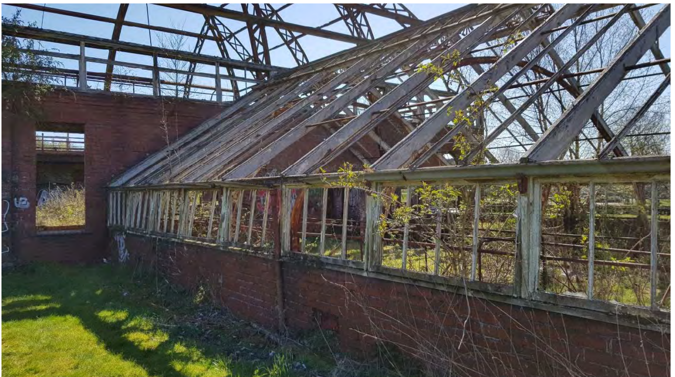
73 – Some movement of wing glazing frames on existing masonry walling
