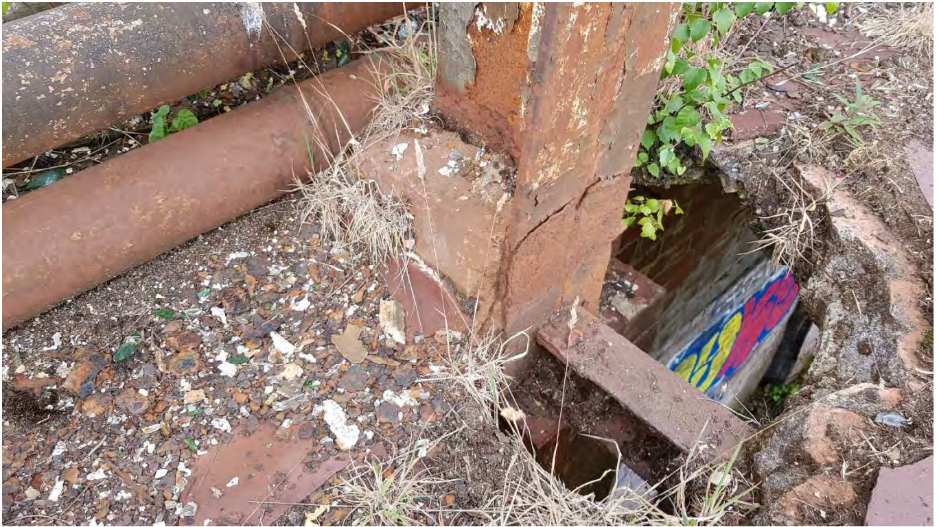
11 – Close-up view at base of main frame showing the steel is intact but has delaminated and needs some attention
