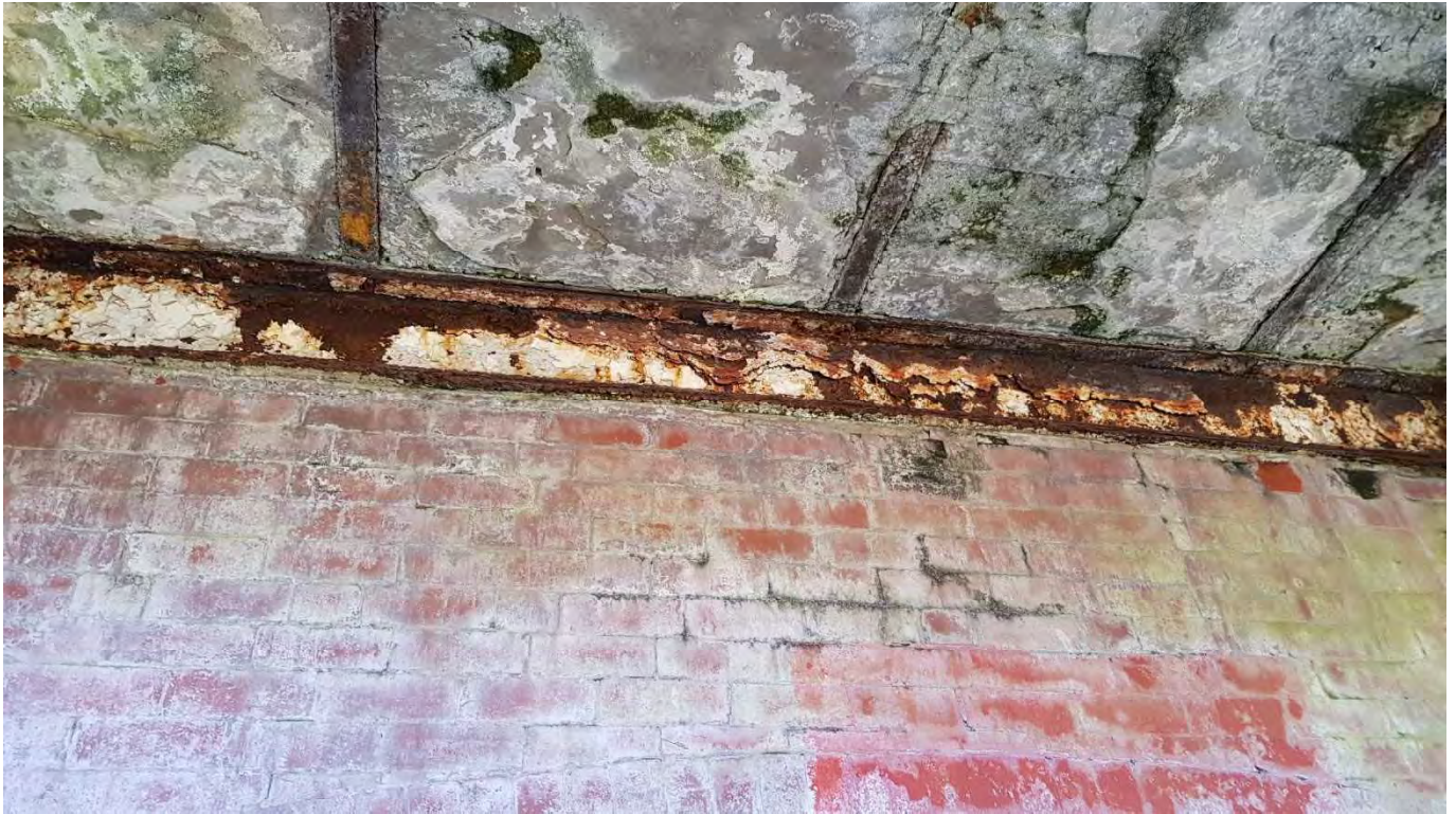
56 – Corroded edge beam with filler joists and main beam needing repainted and potentially repaired
