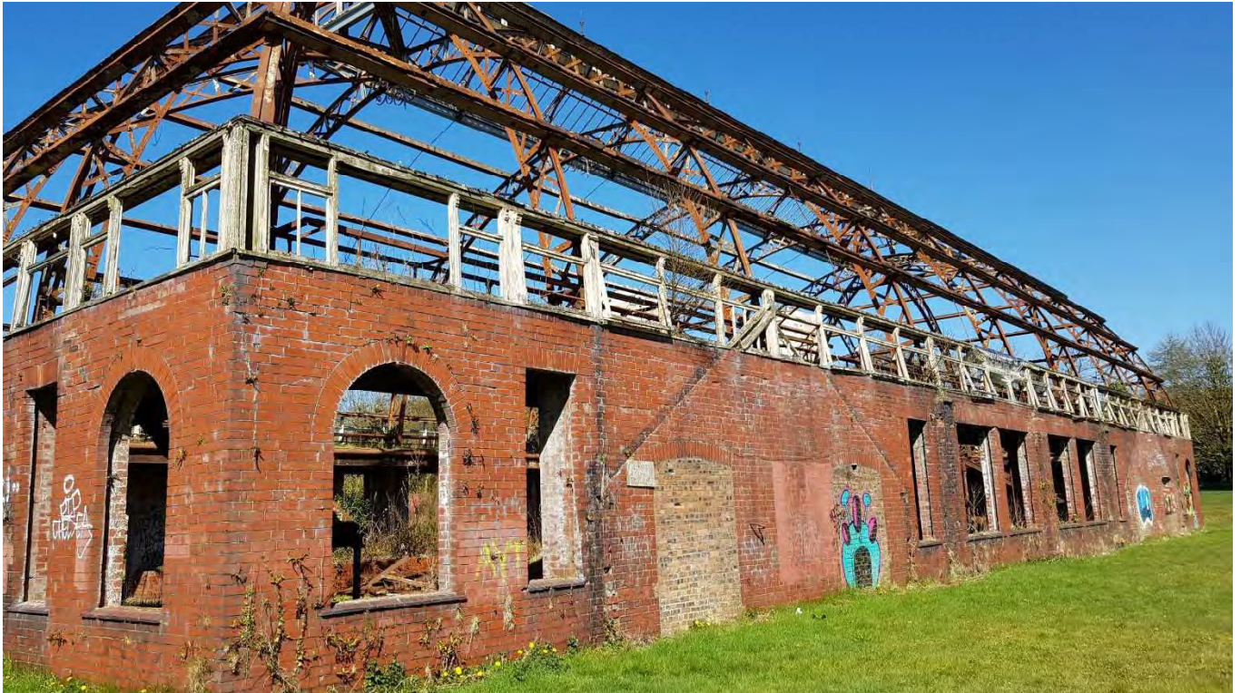
29 – View of east elevation showing previous openings bricked-up and the vestige of eastern glasshouses. Vegetation growth has rooted in the masonry mortar joints and will need to be removed
