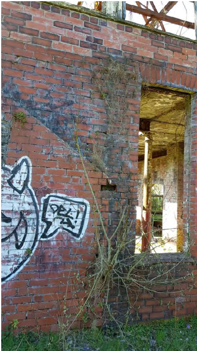
40 & 41 – Vegetation growth is causing severe damage to sections of masonry and removing water ingress and roots to limit water penetration and jacking of masonry is key for any repair
