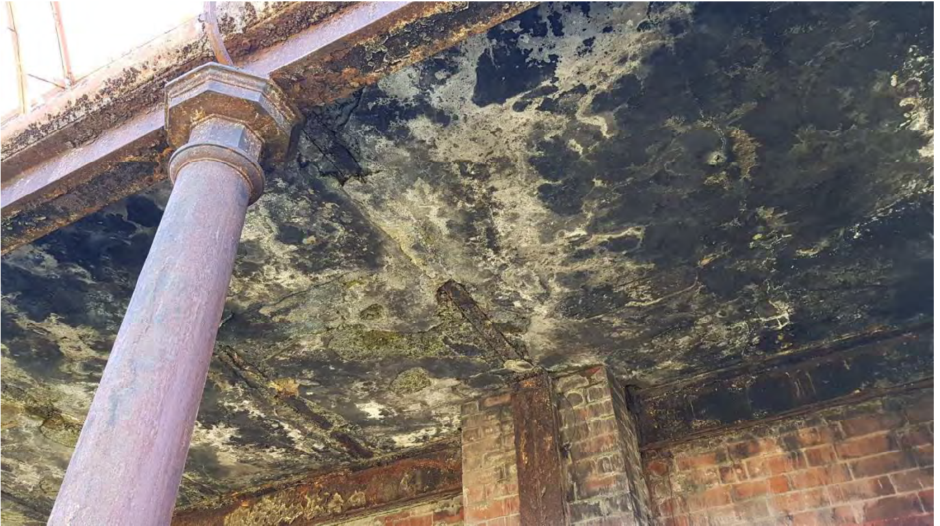
23 – Cast iron column is in good condition but the slab and filler joists will need some attention, as will the main stanchion base half-embedded in the pier
