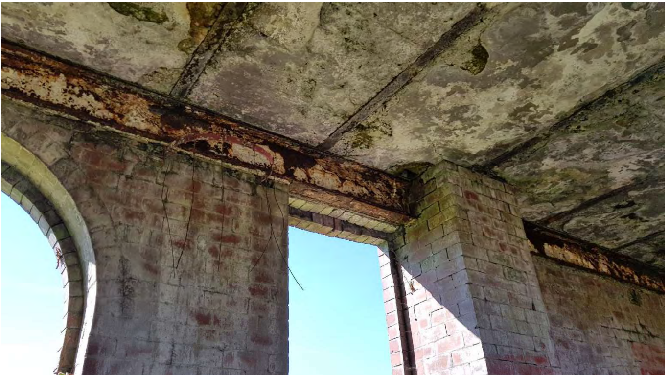
43 – Internal view of internal steel lintel beam showing some deterioration needing re-painted
