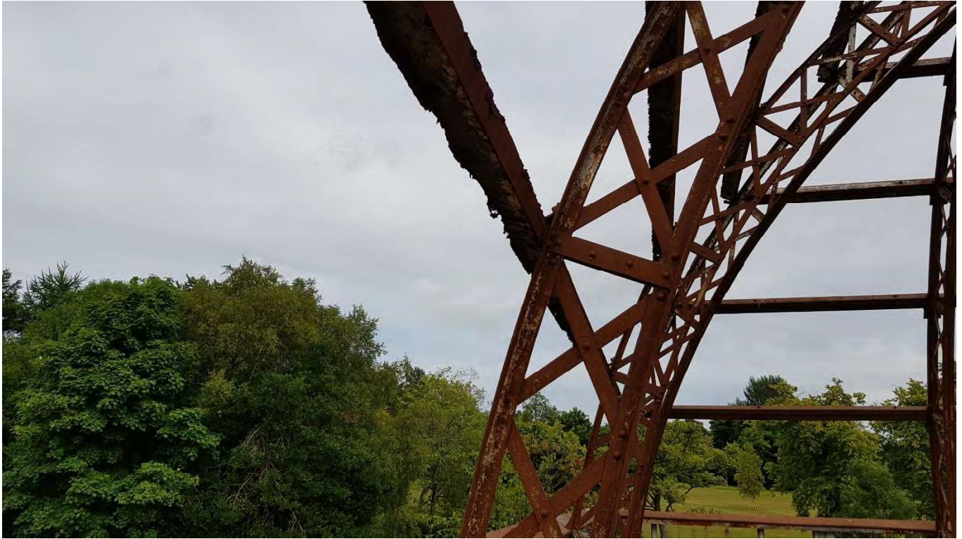
5 – North elevation purlin deterioration showing severe section loss to single purlins on the north and south main elevation frames
