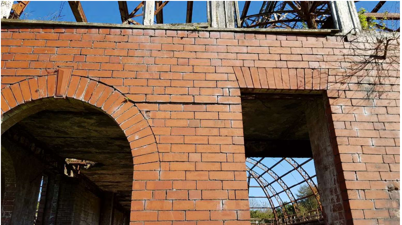
31 – Close-up of some root damage and dislocation of a course of masonry
