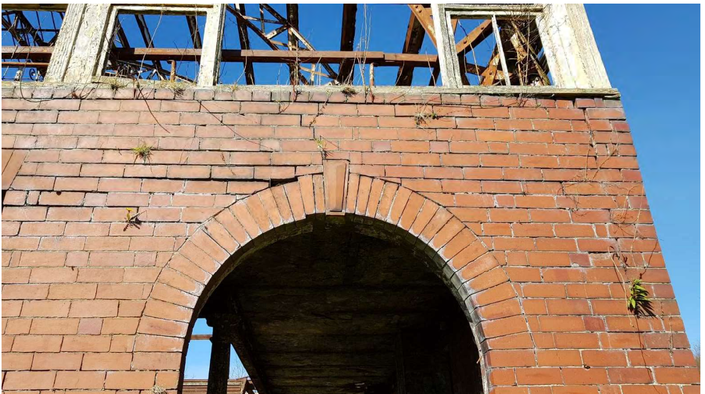
37 – Local arch slip failure due to vegetation growth and some expansion of the upper walling
