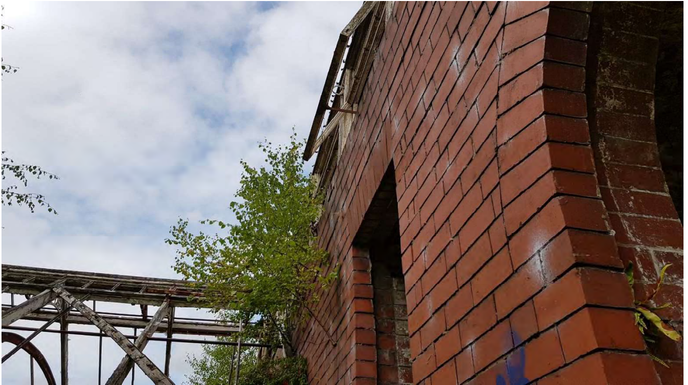
42 – View of south-west upper wall panel showing it 'prying' outwards locally – this will need re-set
