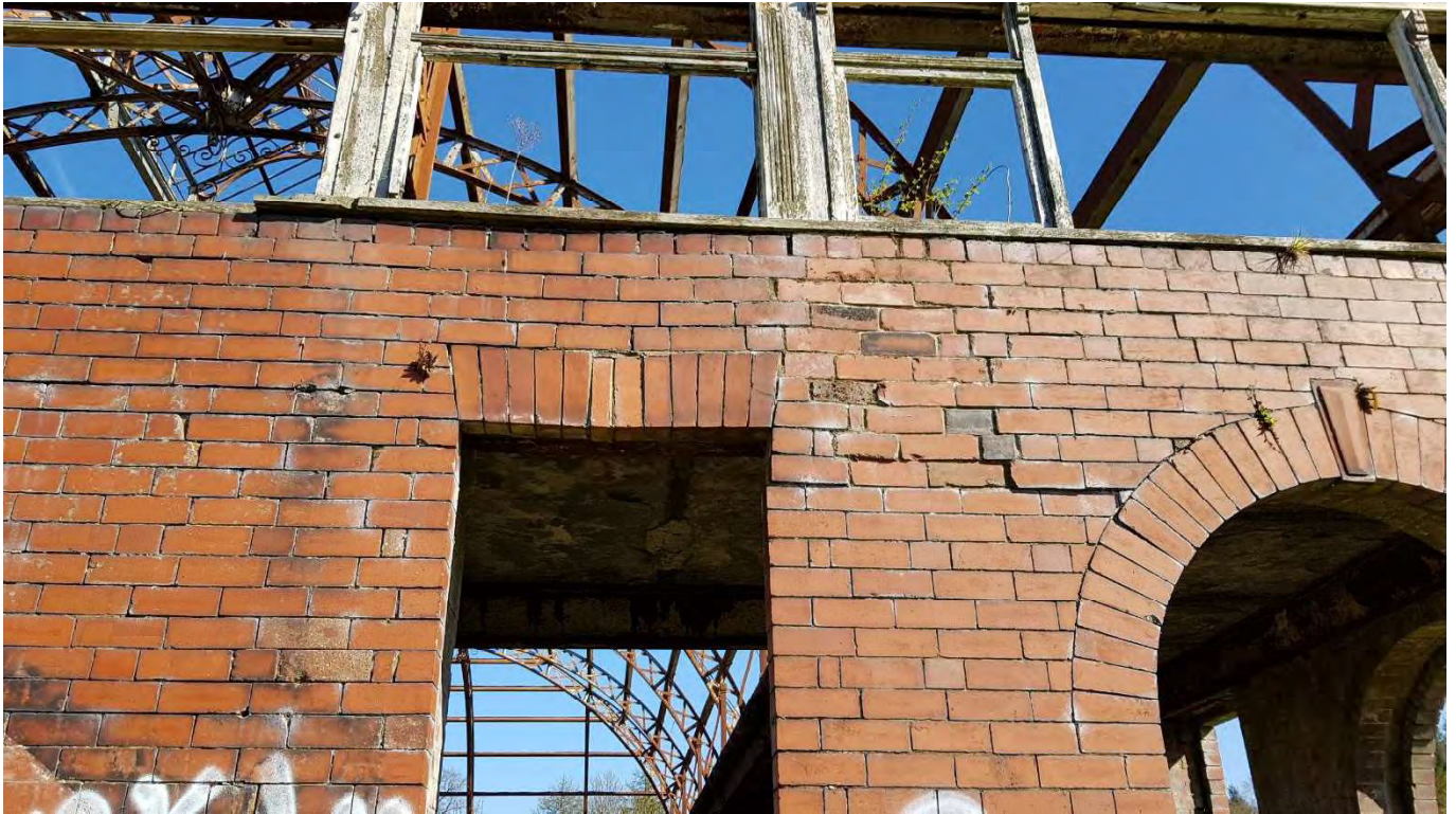
34 – Movement of masonry and failure of flat arch requiring some re-building and repointing
