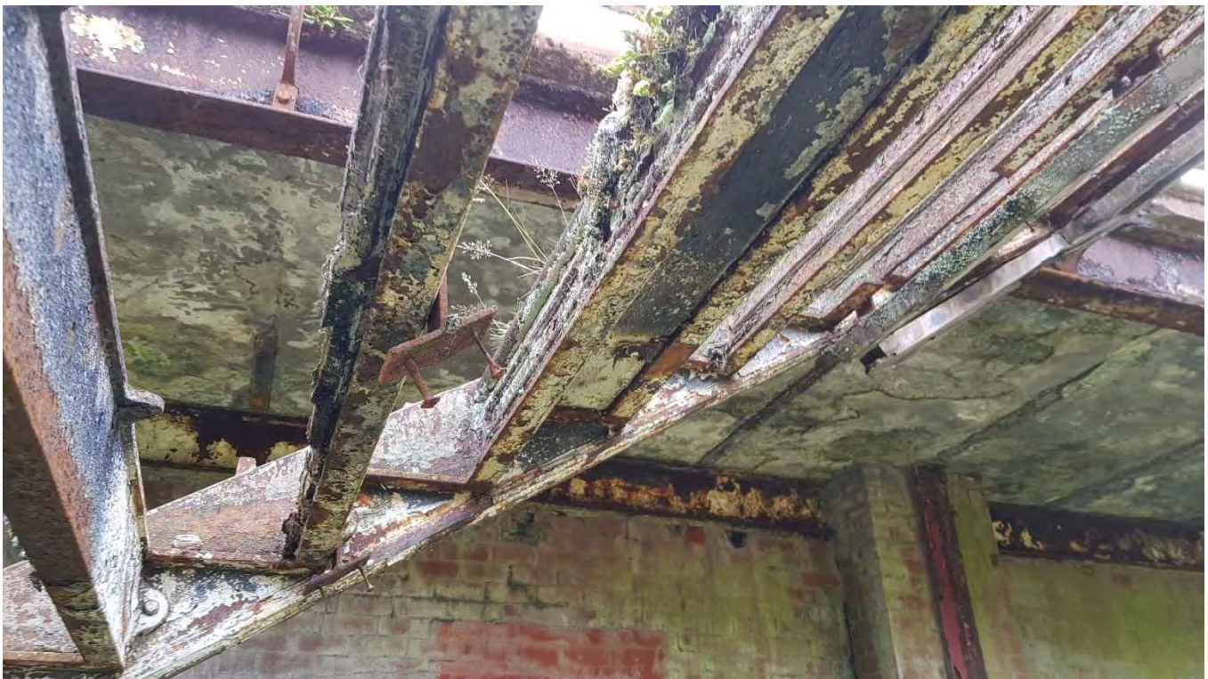
28 – Close-up of steel stairs showing surface deterioration but intact joints
