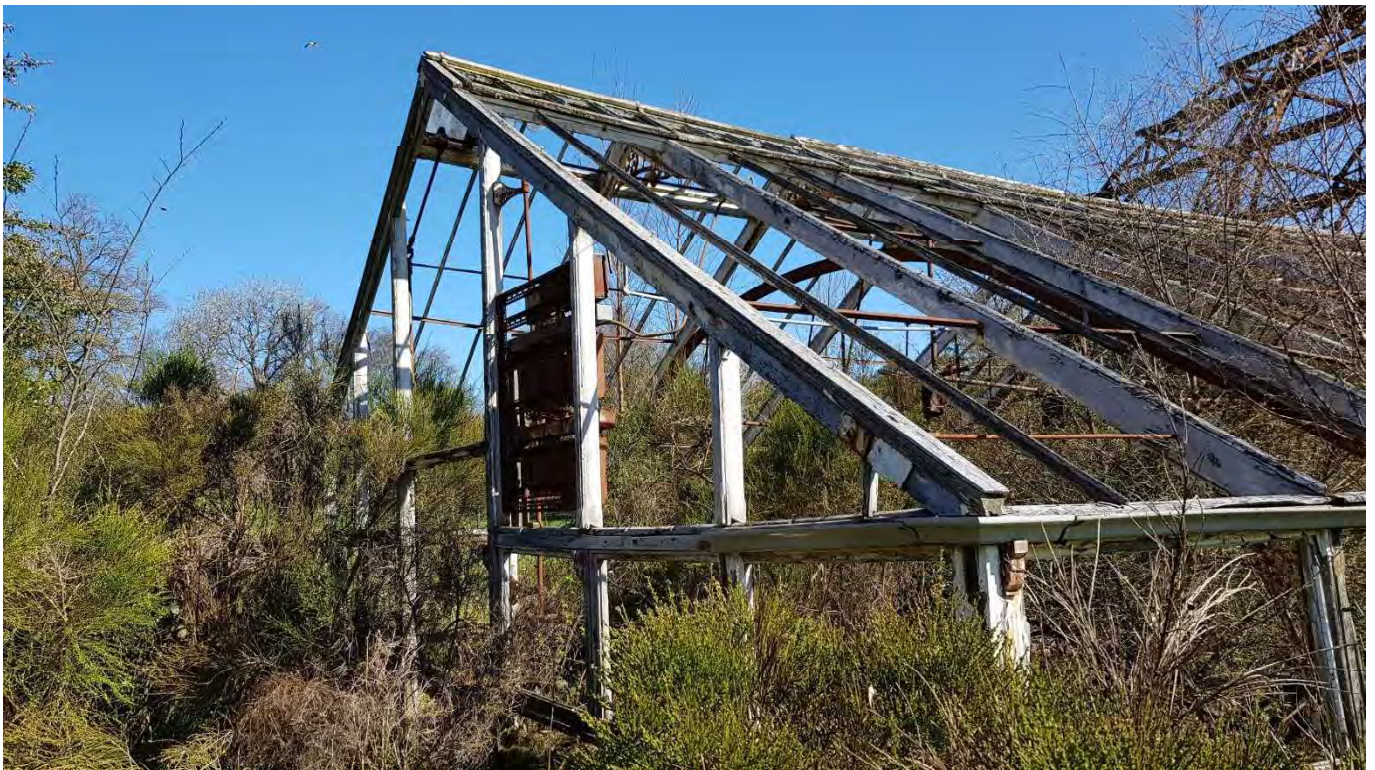
67 – End frame with timber uprights in place and some movement in the eaves beams
