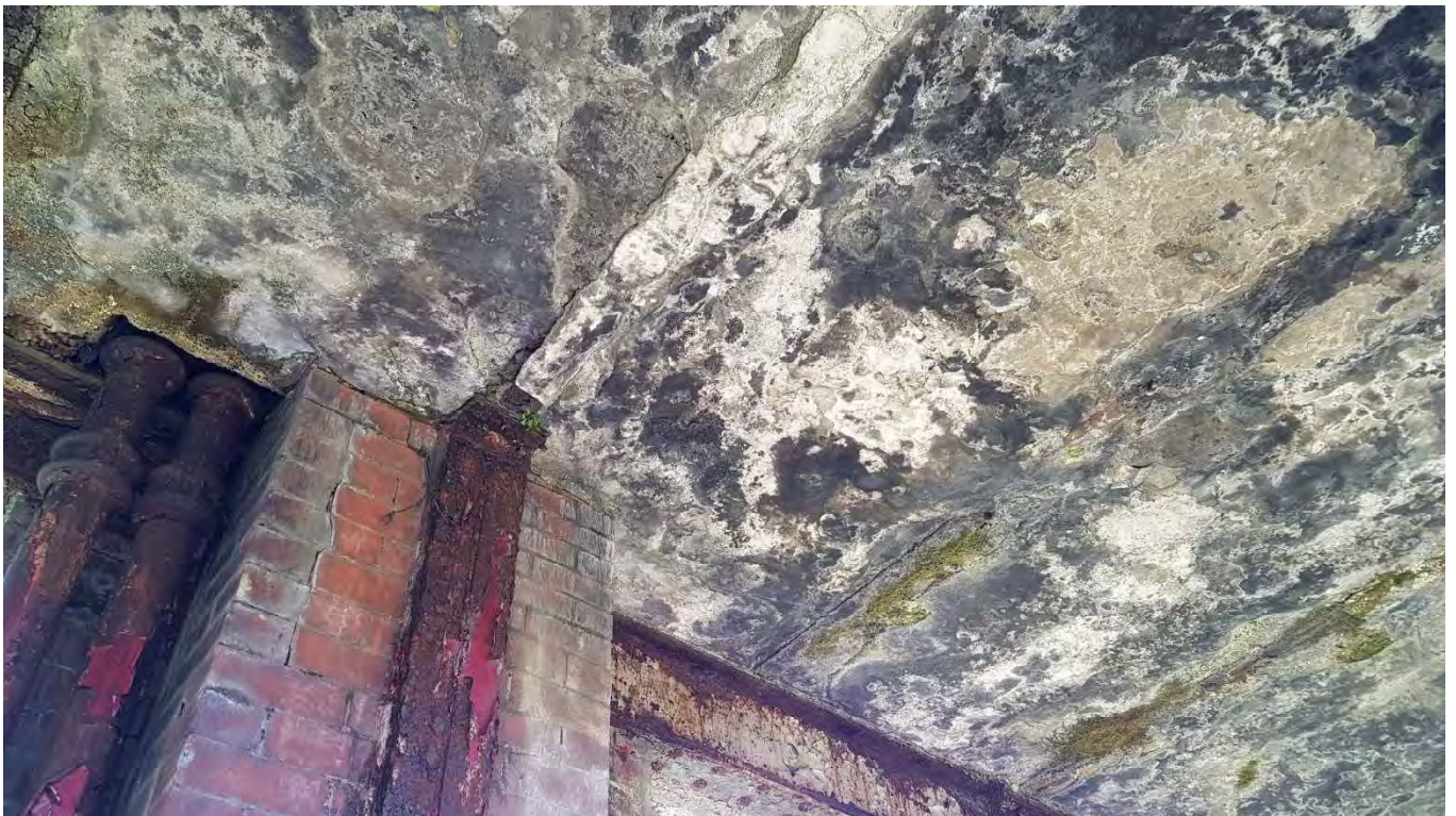
20 – Underside view of balcony at column location showing intact but deteriorating concrete
