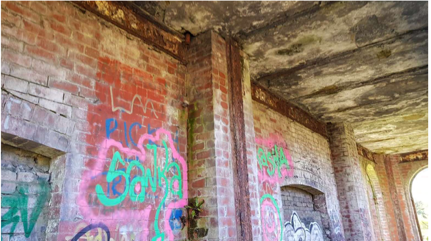
54 – View of internal surface corrosion of embedded stanchion – all steelwork embedded will need to be assessed in due course to determine final repair detail
