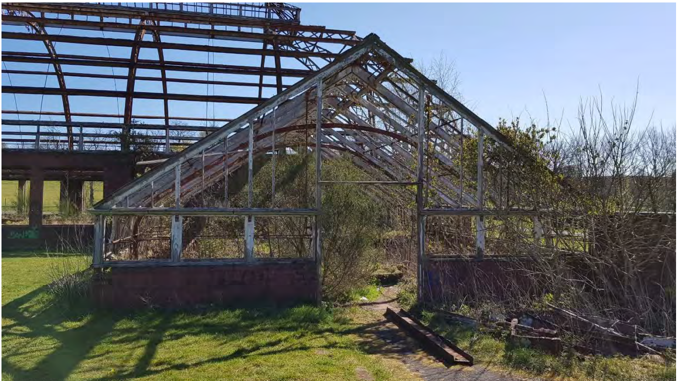
71 – West wall of South Glasshouse showing the internal steel 'hoops' and intact timberwork
