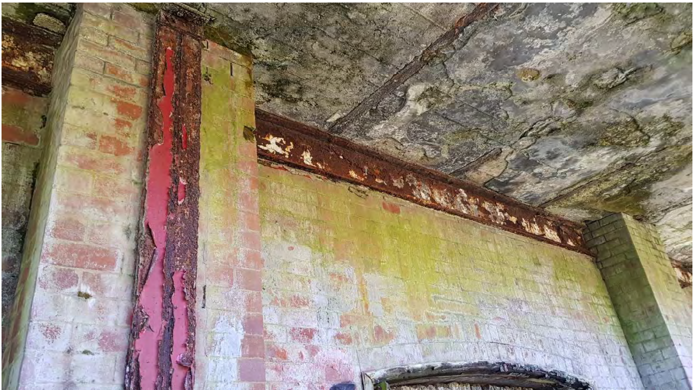
57 – Embedded stanchion with paint still visible
